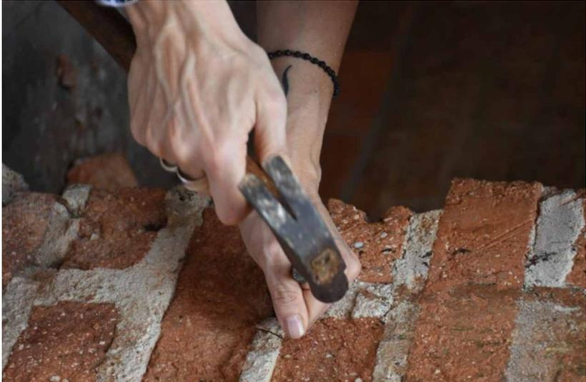
A close-up photograph showing a person's hands using a metal chisel to carefully chip away at the mortar between red bricks in a wall. The person is wearing a black beaded bracelet and a ring. The background is dark, focusing attention on the sampling process. |
